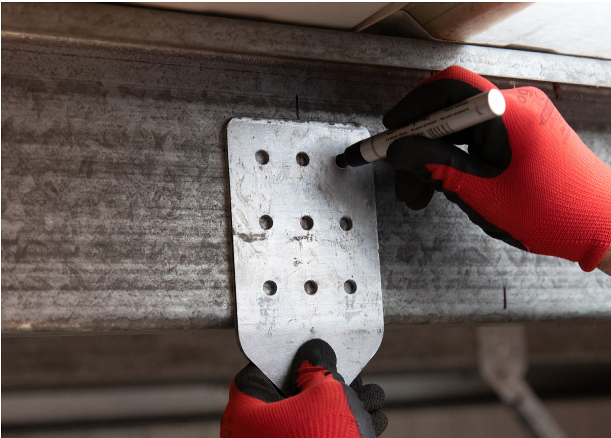
Fig. 1: Incorrect - bracket bends towards you
