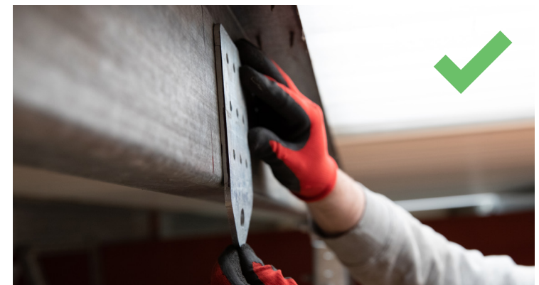
Fig. 2: Correct - bracket bends away from you
