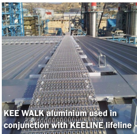
KEE WALK used with integral guardrail
