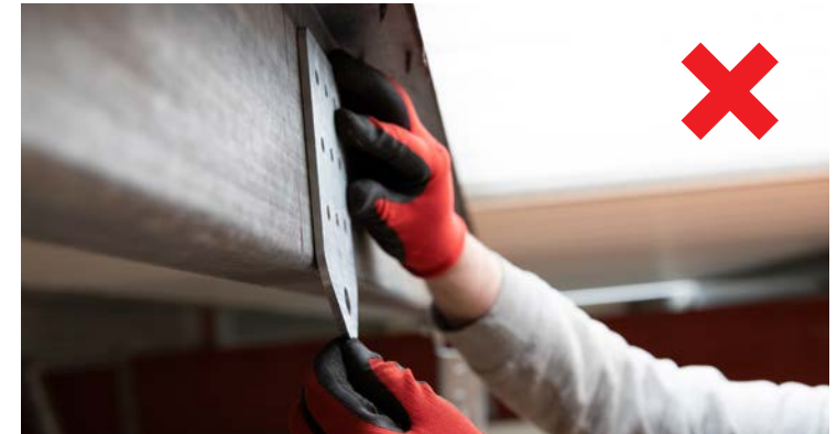
Fig. 1: Incorrect - bracket bends towards you
