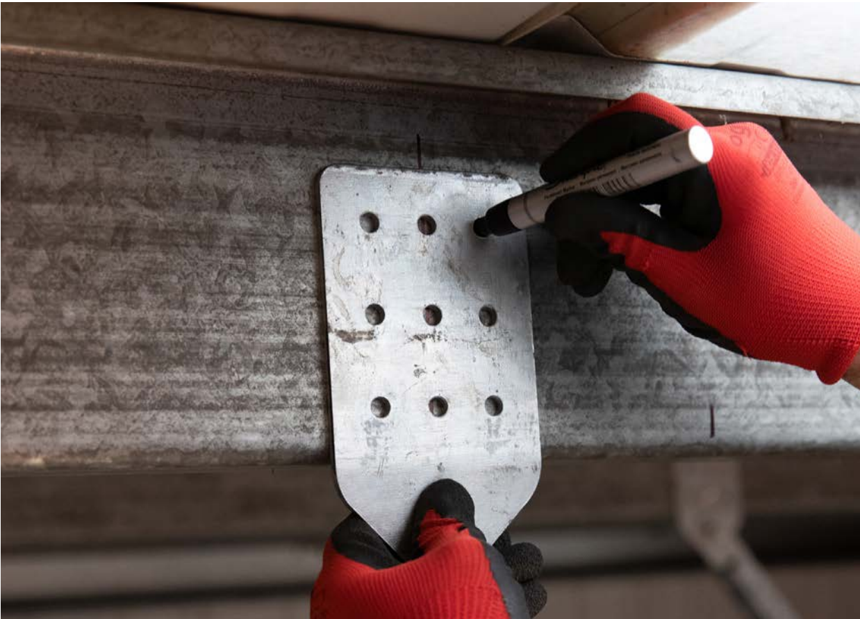
Fig. 1: Incorrect - bracket bends towards you
