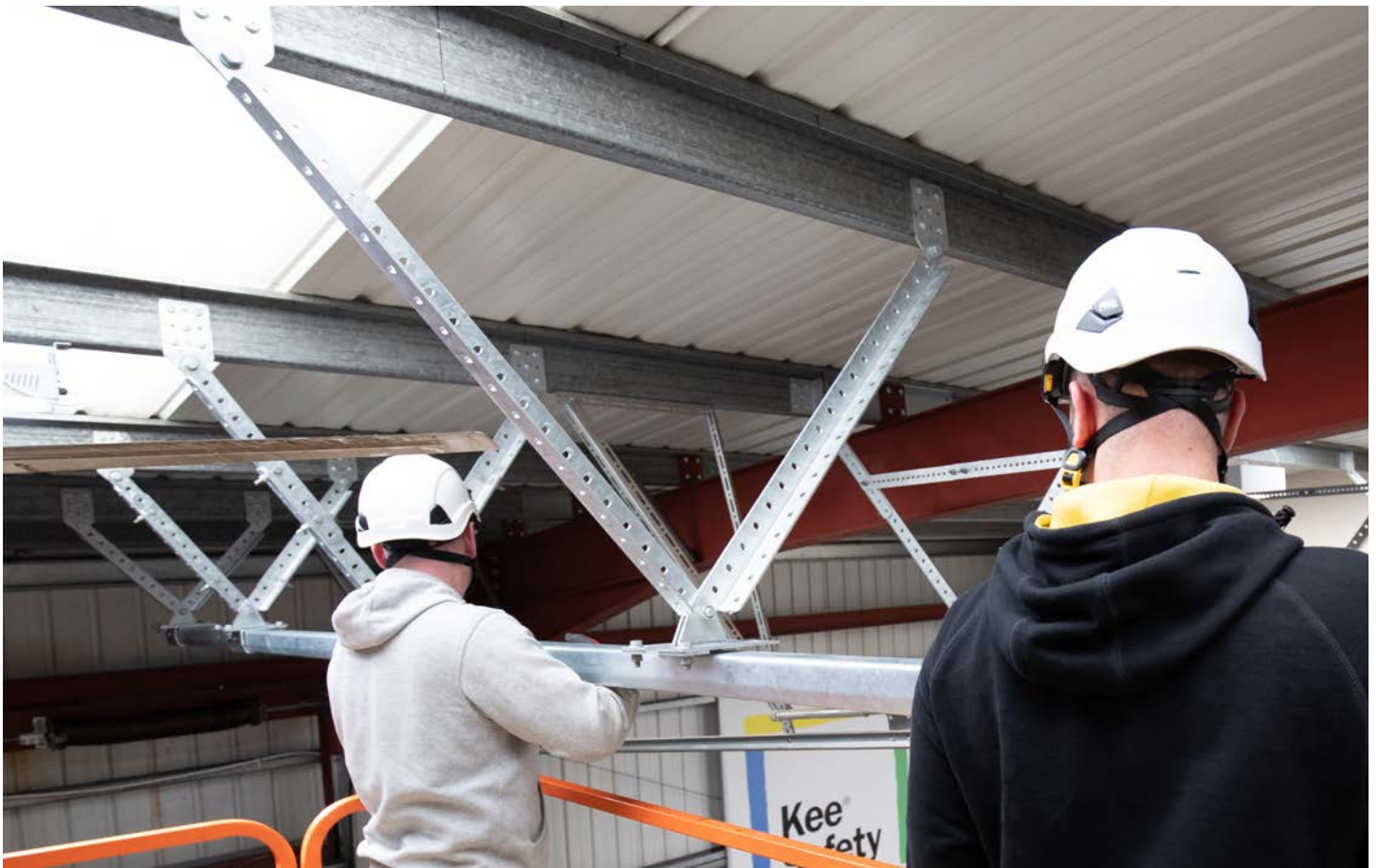
Two installers using an elevated platform secure the rail to the roof infrastructure.
