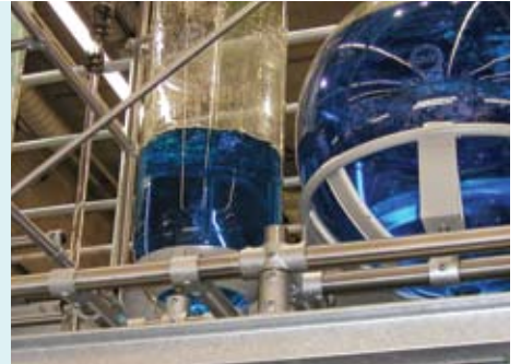
Right: Industrial Process Plant Structures
