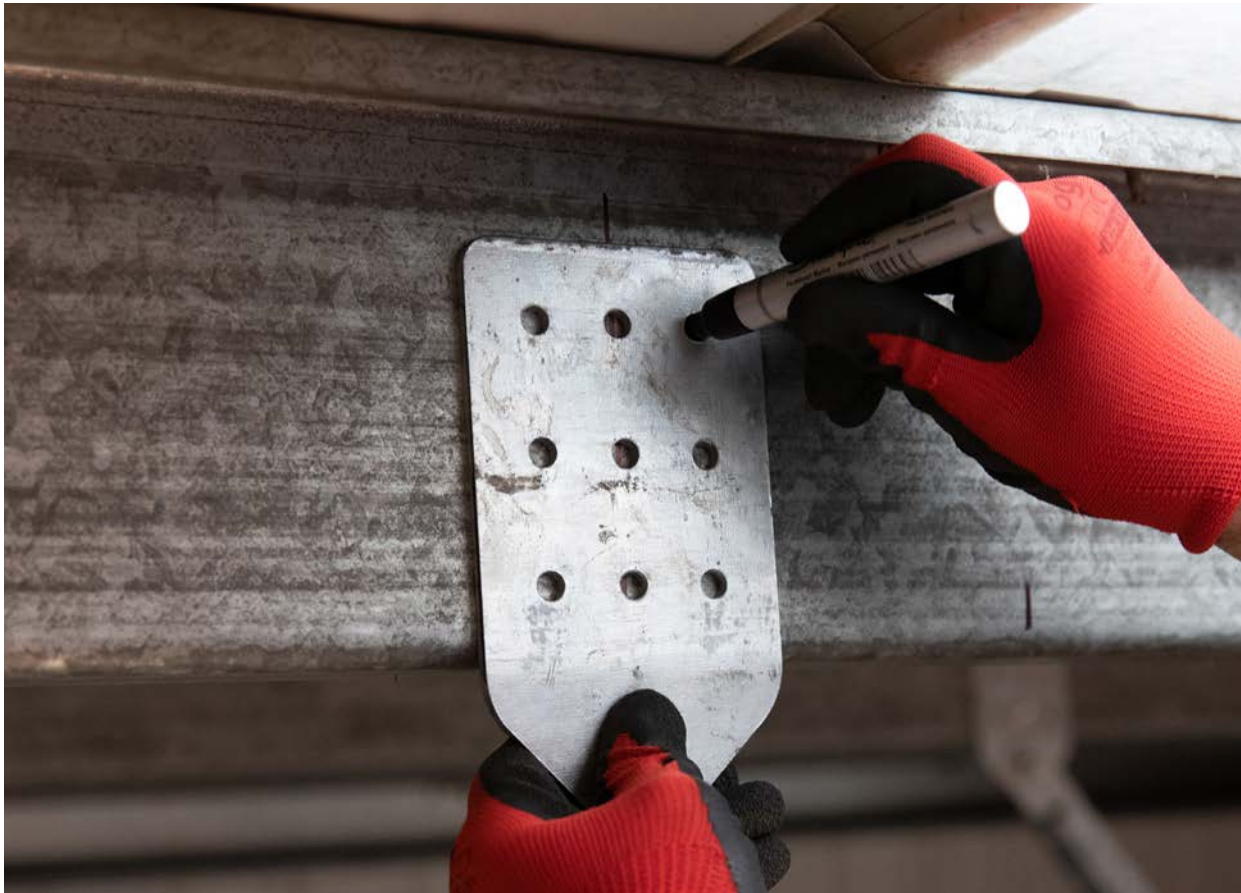
Fig. 1: Incorrect - bracket bends towards you
