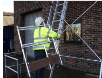
Fig 1 Easi-Dec Ladder spurs.
