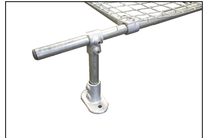
K. Slide 1No. Rail Flange fitting over each end of the exposed tube in the corners of the frame. Carefully align the fitting to ensure it is positioned on the crown of roof sheet.
