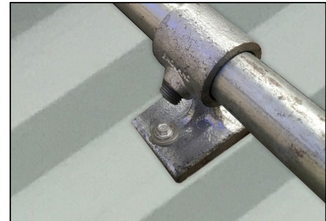
K. Carefully cut 4No. 80mm lengths of sealing strip. Place the Sealing Strip between the 4No Rail Support fittings and the roof structure. Use Self Drilling Screws (SDS55X55G) to attach the screen onto the roofing sheet.
