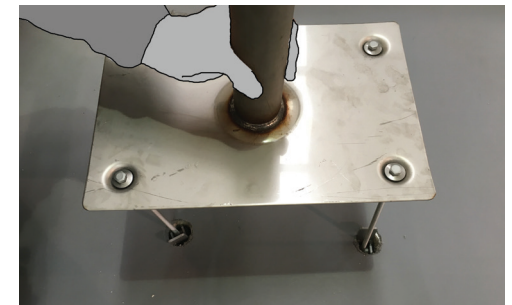
d) Carefully lift the post with fitted toggle bolts attached and offer the toggle bolts (LAKL2TOG4) into the pre-drilled holes through the roof.
