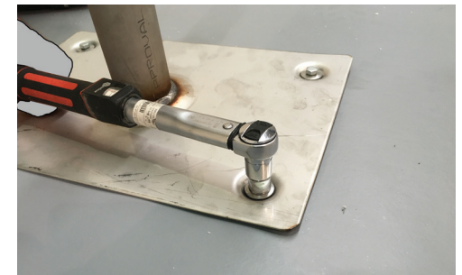
f) Once tightened torque to 8 Nm to ensure they are all fitted correctly. Fit the selected weather proof cawling and complete the required weatherproof detail. (Note:- This may be a specialist roofing contractor).
