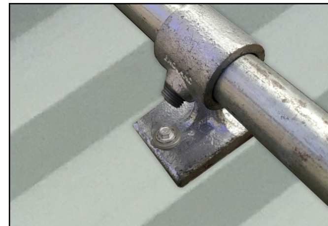
K. Carefully cut 4No. 80mm lengths of sealing strip. Place the Sealing Strip between the 4No Rail Support fittings and the roof structure. Use Self Drilling Screws (SDS55X55G) to attach the screen onto the roofing sheet.
