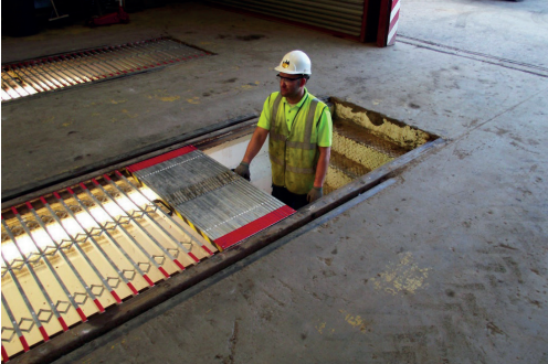
Open end of cover to access the pit via steps.
