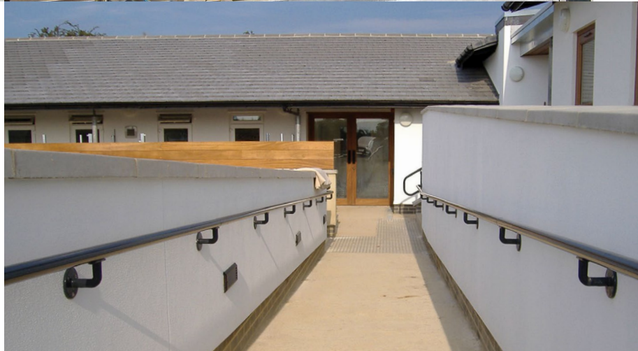
Right: ADA Compliant Railing for Access Ramps
