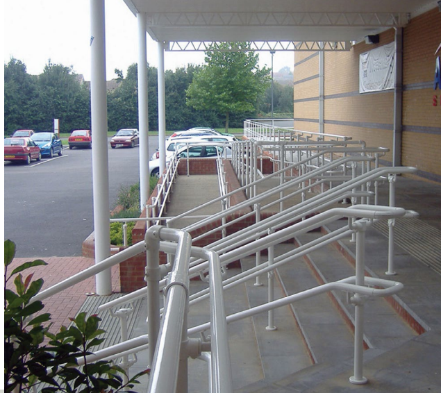
Right: ADA Compliant Railing for Public Access
