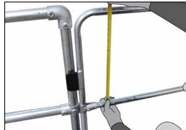
N. Use a measuring tape to ensure gap between top rail and mid rail is no more than 470mm. Adjust if necessary.
