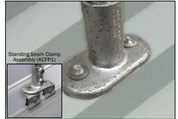
L. Carefully cut 2No. 120mm lengths of sealing strip. Place the Sealing Strip between the 2No. Standard Rail Flange fittings and the roof structure. Use Self Drilling Screws (SDS55X550) to attach the screen onto the roofing sheet. NB If attaching to standing seam roof use KCFP1 clamps to connect to the standing seam and bolt the 62-5 fitting to the KCFP1 clamp as shown in the diagram.
