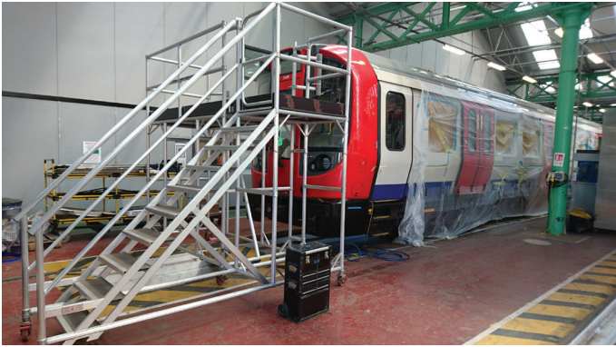
Build depots and maintenance sheds
