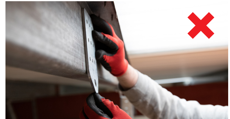
Fig. 1: Incorrect - bracket bends towards you
