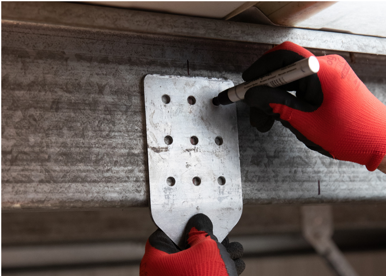
Fig. 1: Incorrect - bracket bends towards you
