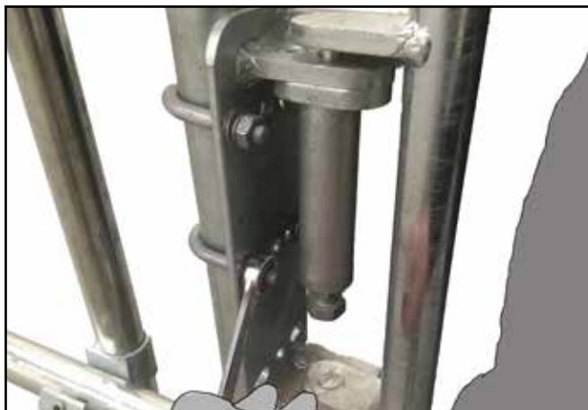
C. Pass U-Bolt around the support leg/structure and feed through the middle holes of the fixing plate. Using a spring washer, flat washer and nut to connect the U bolt to the fixing plate.
