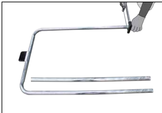
I. Using a hacksaw or similar, carefully cut through the top, bottom tubes and mid rail as shown. For galvanised assemblies, spray with Galvafruid or similar to prevent corrosion.
