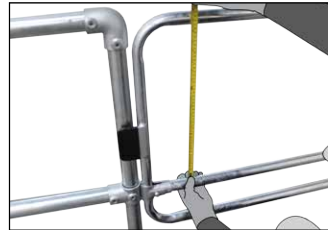
Q. Use a measuring tape to ensure gap between top rail and mid rail is no more than 470mm. Adjust if necessary.
