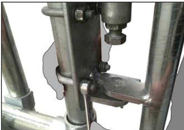
D. Pass U-Bolt around the support leg/structure and feed through the bottom holes of the fixing plate. Using a spring washer, flat washer and nut to connect the U bolt to the fixing plate.
