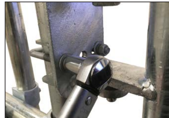
E. Torque all nuts/U Bolts to 39Nm using the 13mm or 17mm socket and torque wrench. Repeat steps A-E for right hand side gate.
