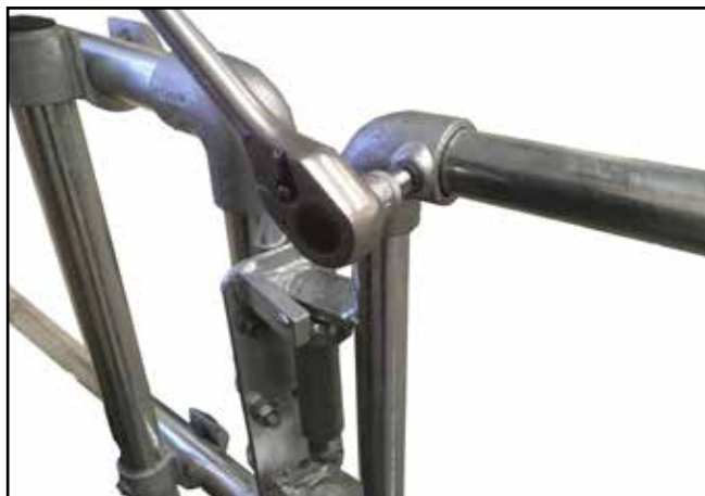
J. Carefully re-position the gate top and bottom tubes into the cast fittings. Use a spirit level, to ensure the gate is level. Tighten the cast fittings grub screws using a hex head socket. Using the torque wrench ensure the castings are torqued to 39Nm. Repeat steps G-J for right hand gate.
